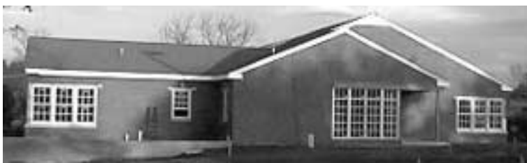
The façade of the new Franconia Township Police Department as it nears completion.
