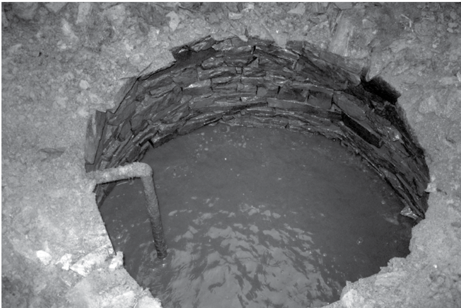
This well was unearthed during the Erie Road construction.
