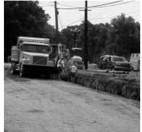
Intersection realignment work being done at Godshall Road and Route 113.
