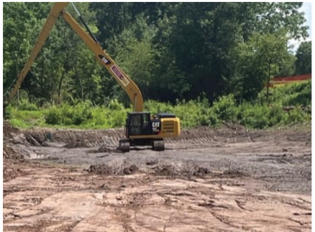
Work being done on the new bio-retention area at Enos B. Godshall Park
