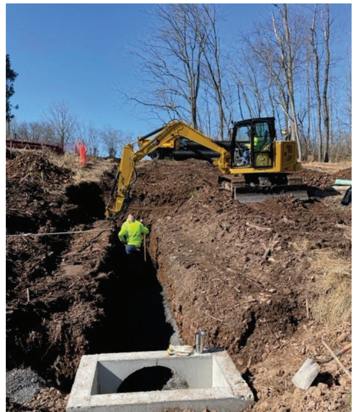
A new storm inlet is installed at Enos Godshall Park
