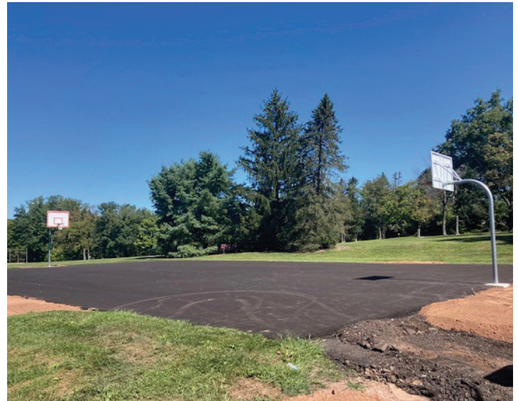
Branchwood Park basketball court under construction
