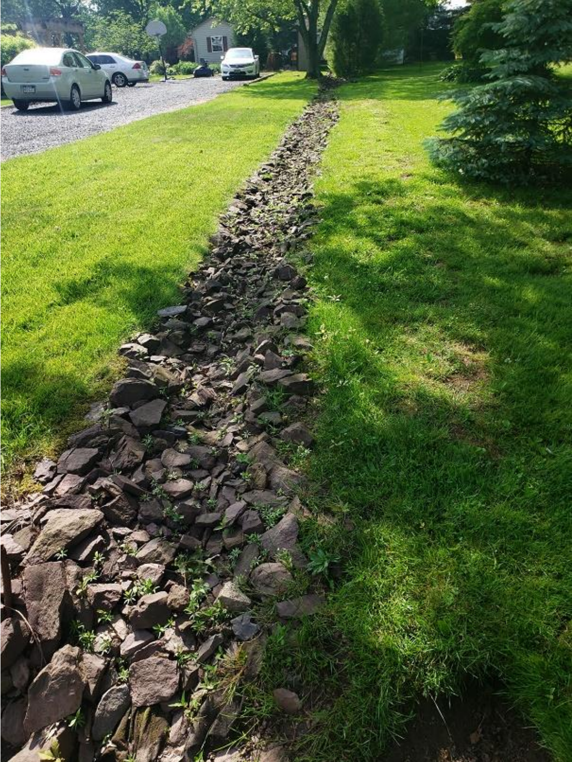
Drainage ditch originating from the property of 274 Telford Pike. This ditch discharges into the ditch on Telford Pike.
