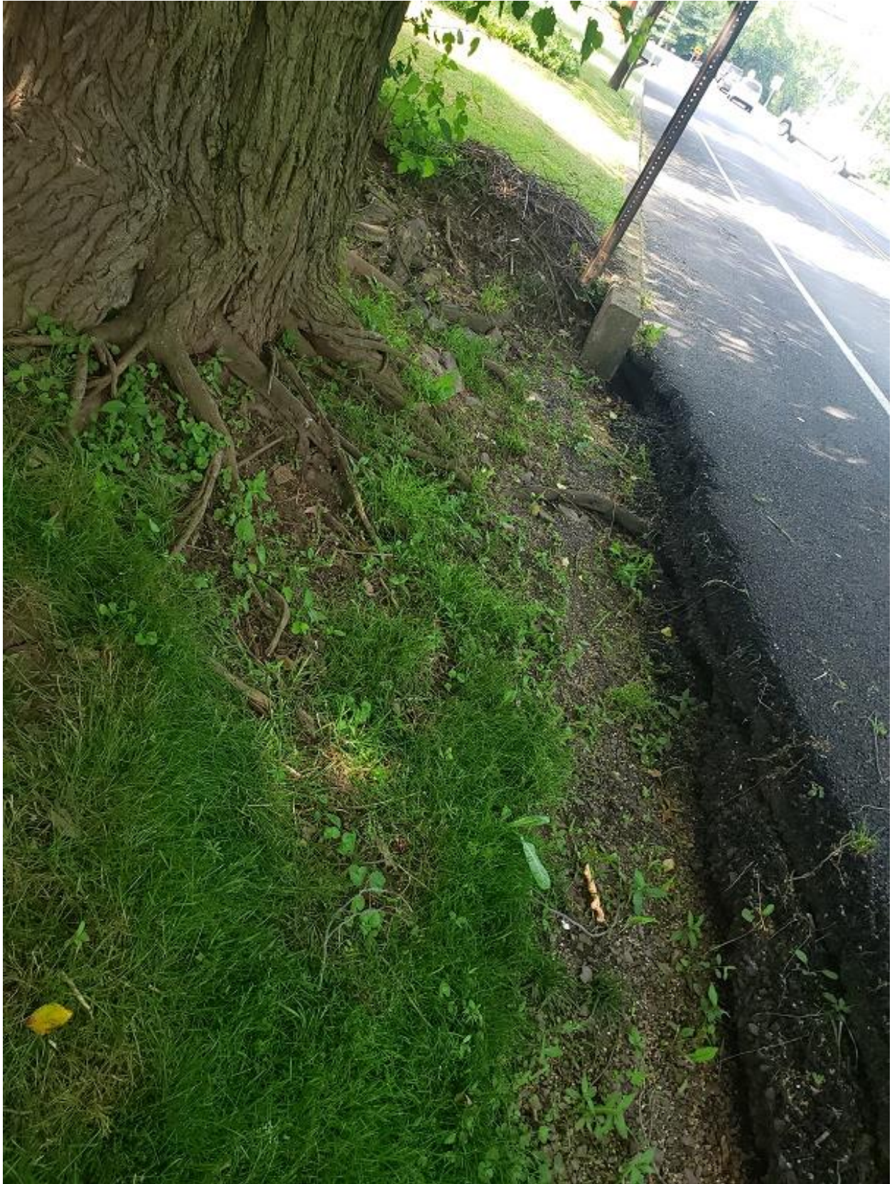
Beginning of ditch along Telford Pike.
