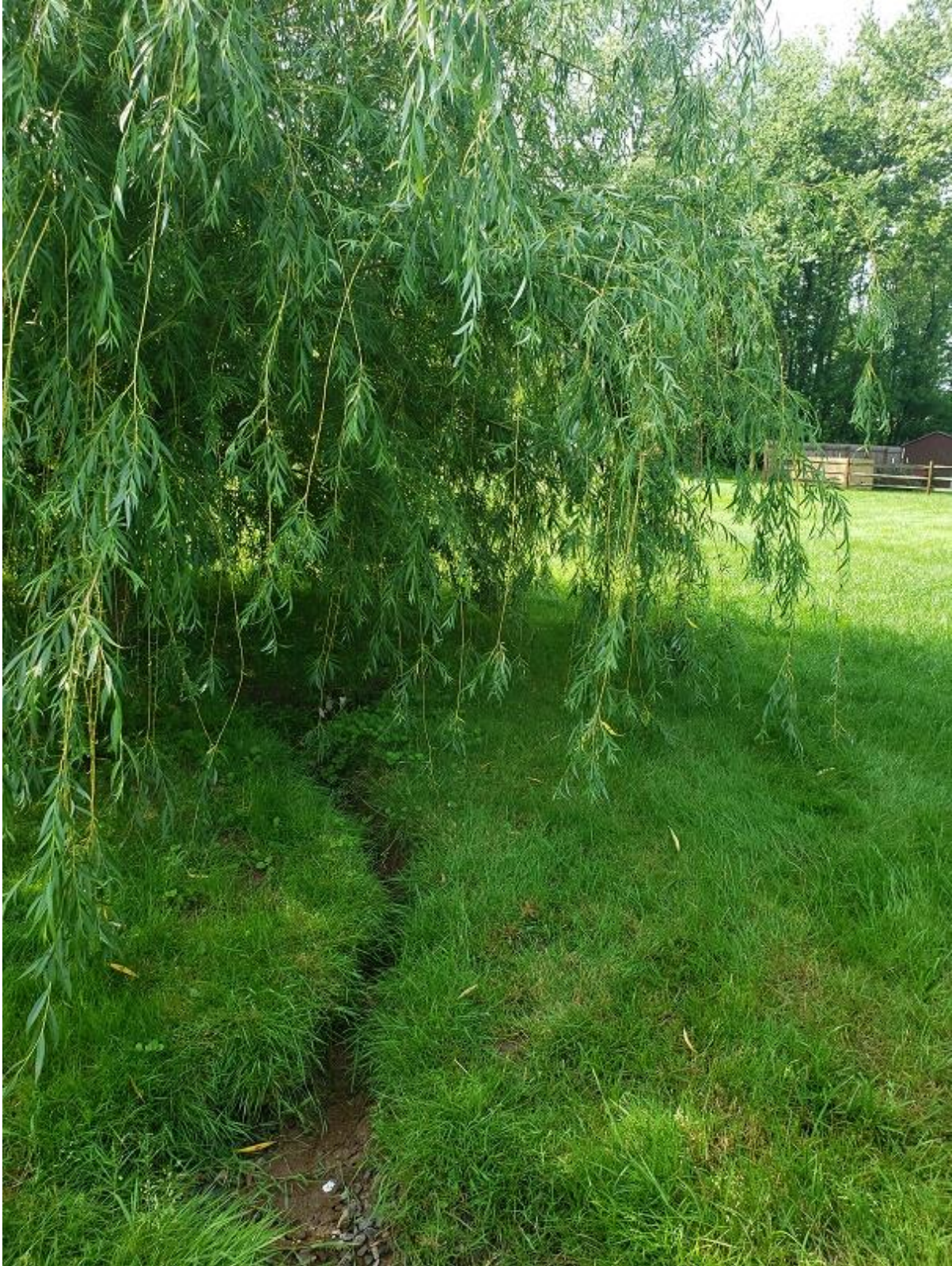
Willow tree behind 511 Bergey Rd. Ditch is beginning to erode.
