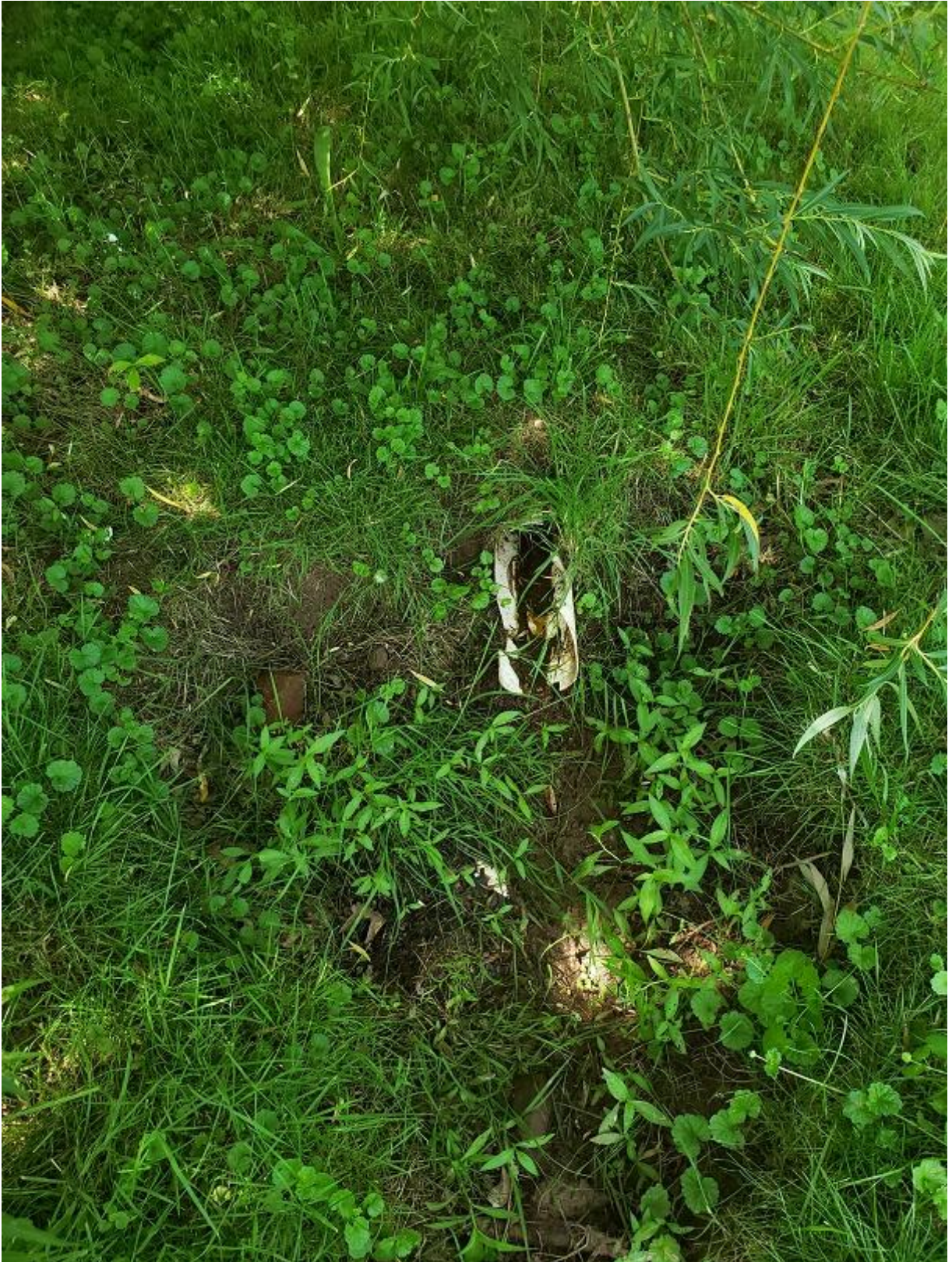
Discharge pipe near Willow Tree.
