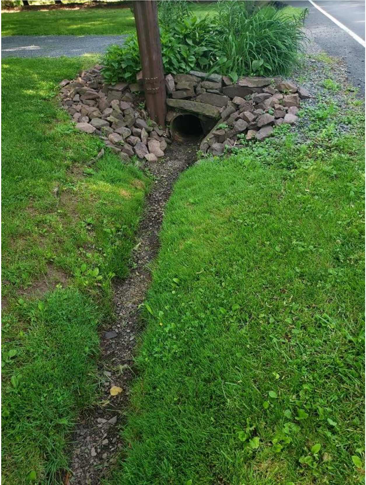
Ditch continues under driveway through culvert.
